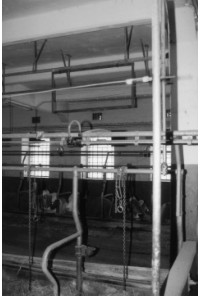
Fig. 5 Arrangement and construction of the fly-catching frames (Test 1).
